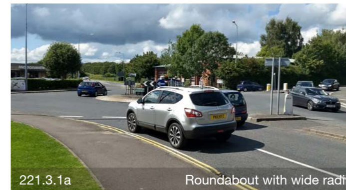
221.2.2 Wide corner radii to support HGVs
